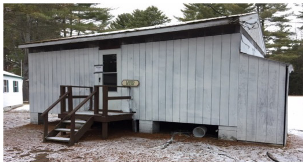
Student Restrooms (left)
